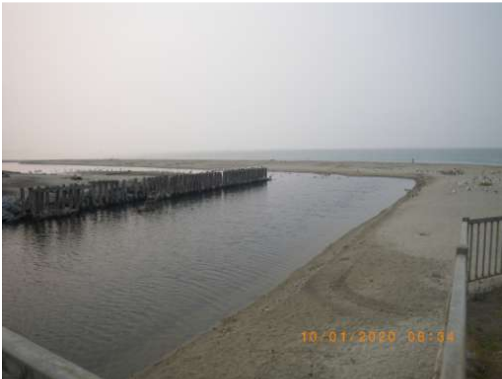
Lower Aptos Estuary with valuable habitat around pilings, looking downstream. 1 October 2020.
