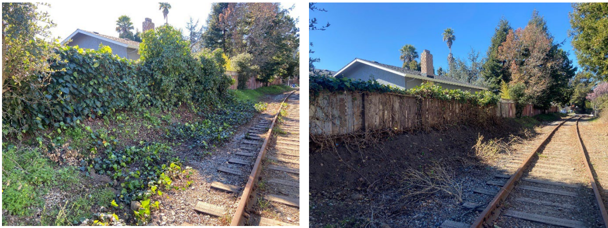
Figure 3 - Before and after at MP 15.15
