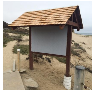
Completed kiosk with protected enclosure
